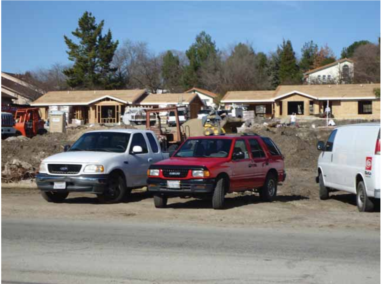
New Single Family Homes Under Construction, 935 - 949 Creston Road
