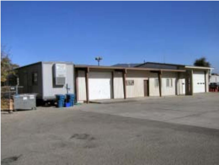
Exterior view of station and current modular building (sleeping for 2)
