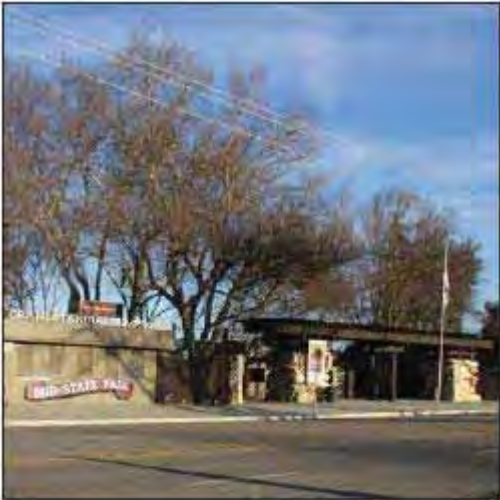
Paso Robles Event Center main entrance
