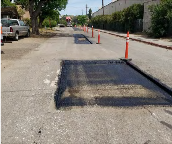
Digout Areas Prepared for Paving
