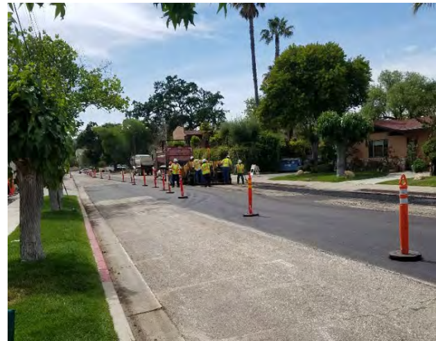
Crew Working Their Way Down the Road
