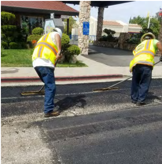
Crew Raking Hot Asphalt
