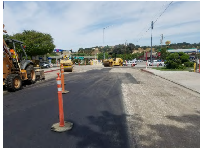
Rollers Compacting the New Asphalt
